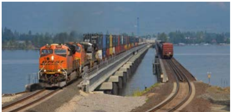
Old and New bridges. Lake Pend Oreille, ID, east of Spokane, WA.
